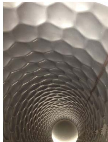
Fig.(3) structure segment from inside
