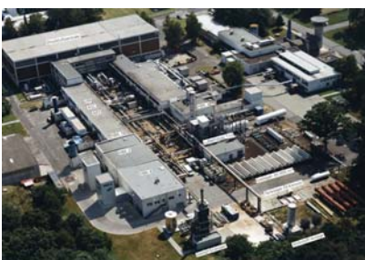
Combustion chamber and compressor test center in Cologne
